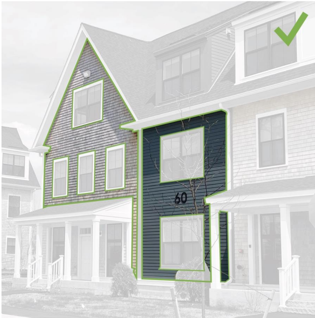
Figure 8: Example of a facade that uses only two materials, including cedar shakes
