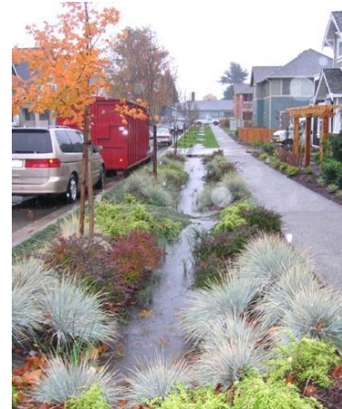
Figure 21: Bioswale
